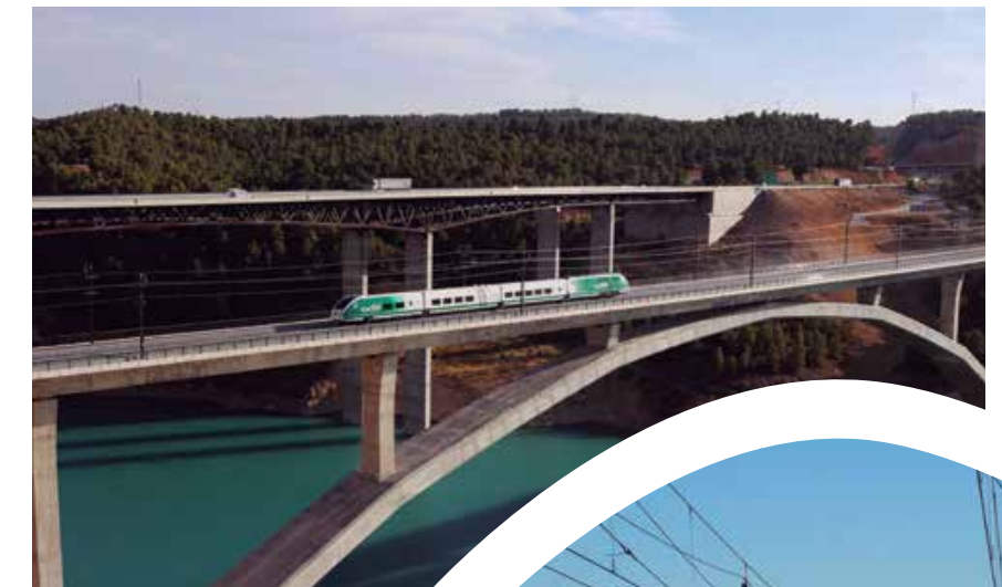
Above, the Contreras viaduct, with the largest concrete railway arch from Europe (261 m of light). It is located in the LAV Madrid-Valencia. On the right, the Sant Boi viaduct.
